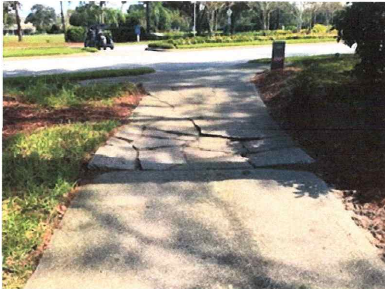
Oak and other trees have cracked and upended the cart paths in several locations
