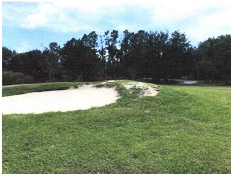
Taking out the hump from the practice bunker is an example of prior shaping would have helped prior to installing sand and a perimeter of new sod would have been recommended to ensure the integrity of the bunkers
